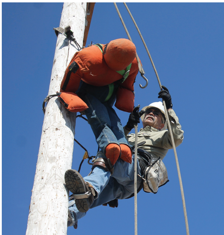
Cotton Electric Journeyman Lineman Terry Turner completes annual pole top rescue training. Photo by Danielle Quickle.
